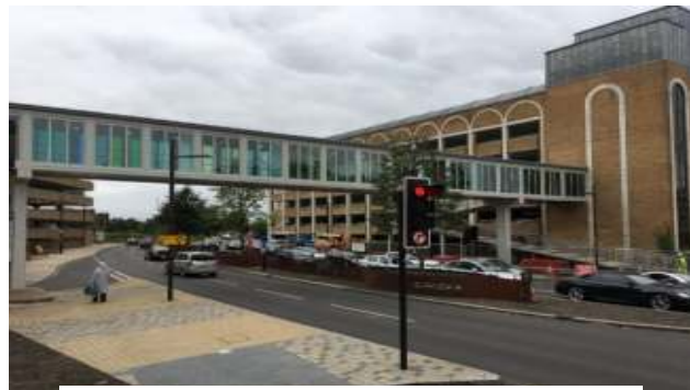
Figure 3.3: Queensgate Footbridge Refurbishment
